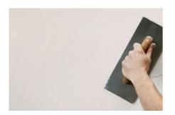
**14.** The ReductoClip System is then ready for standard plasterboard finishing. A plaster skim finish is most common but heavy duty backing paper can also be used.
